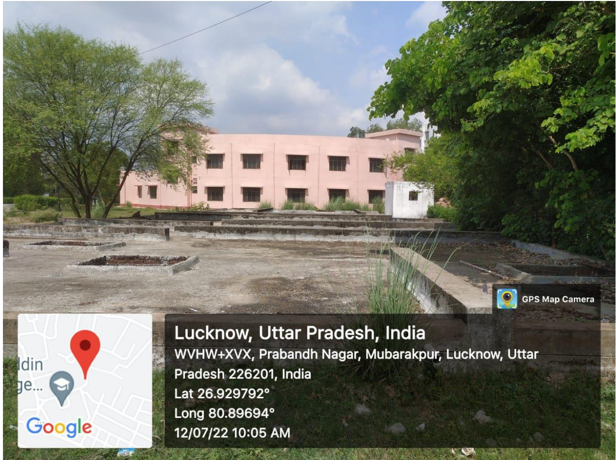
Figure: Underground tanks for water storage for emergency and fire fighting
