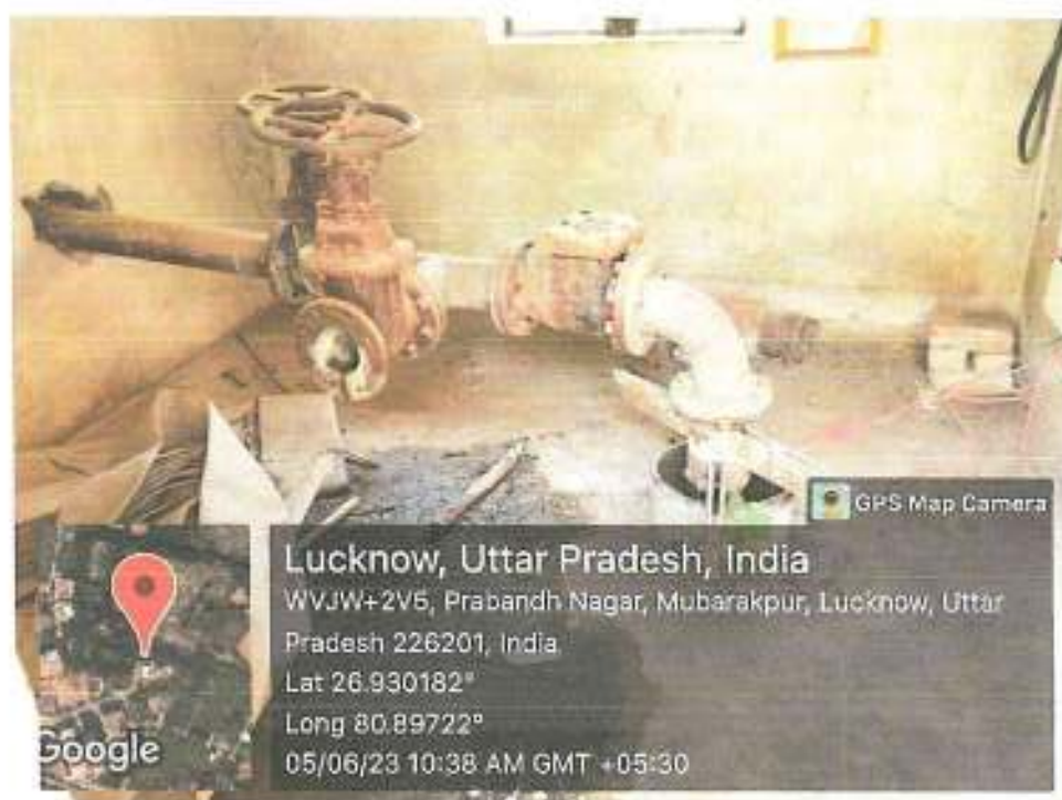
Submersible pump of 10 HP at KMC Language University, Lucknow
