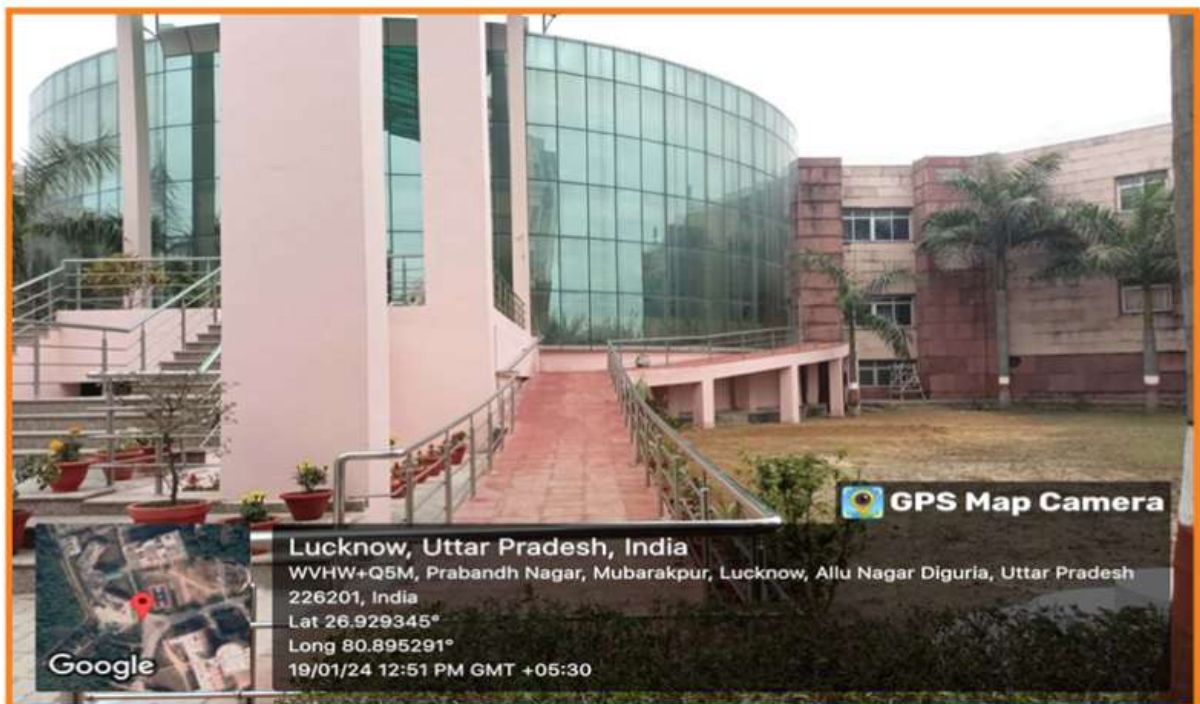
The incorporation of an inclined plane within the Acharya Narendra Dev Administrative Building to ensure accessibility of building for individuals with mobility challenges.
