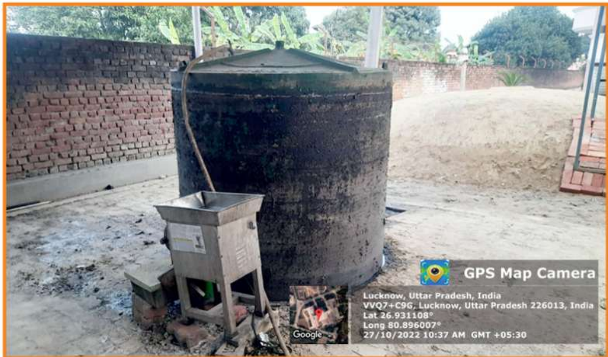
Bio Gas Plant in the University which provides a good amount of cooking Gas which is used in Mess of University Hostel
